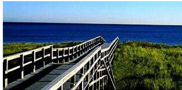
Figure 2: Access across Dune
